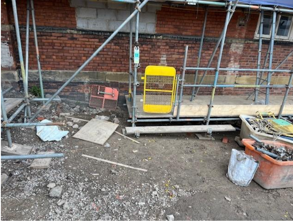
P55 – West Elevation sub-floor (no basement)
