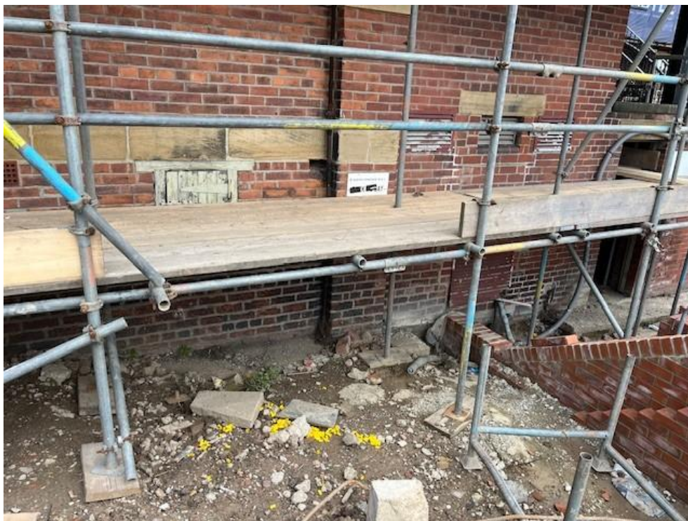
P54 – West Elevation Plant Room
