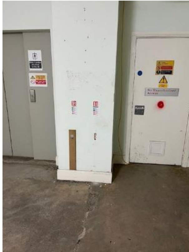
P66 – Circulation Area 02, Wall solid pillar
