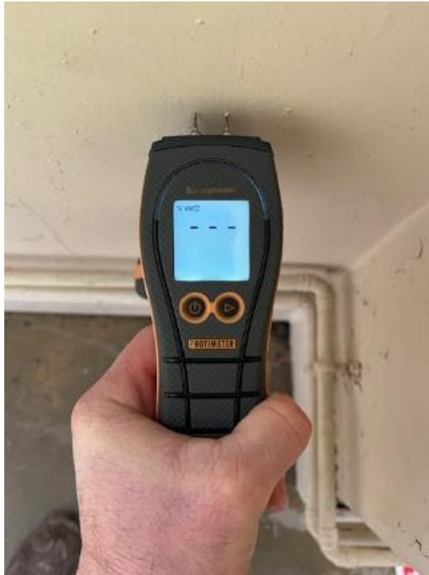
P6 – Store Room, no moisture content recorded
