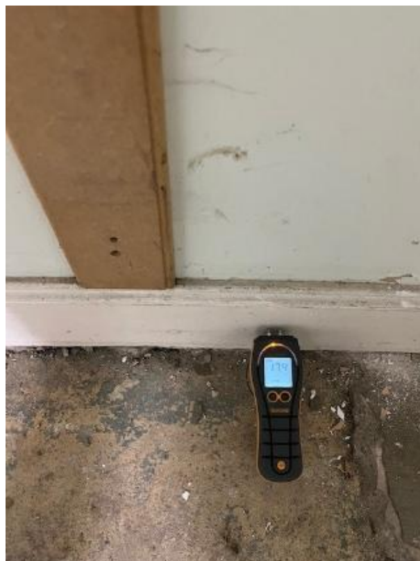
P67 – Circulation Area 02, Wall skirting 17.4%
