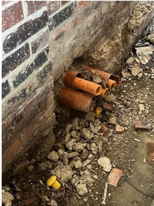
P14 – East Elevation services penetration
